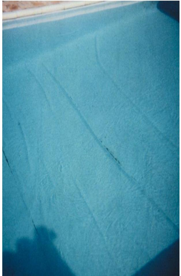
In the picture on the right, the presence of large folds indicates that significant quantities of water are present behind the liner. In effect, the liner is “floating”. There may be leaks at the joints between liner and water inlets or outlets, or maybe there is a ground-water problem.
